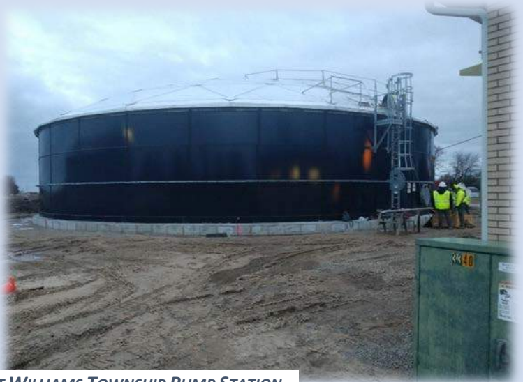
NEW 500,000 GALLON STORAGE TANK AT WILLIAMS TOWNSHIP PUMP STATION
